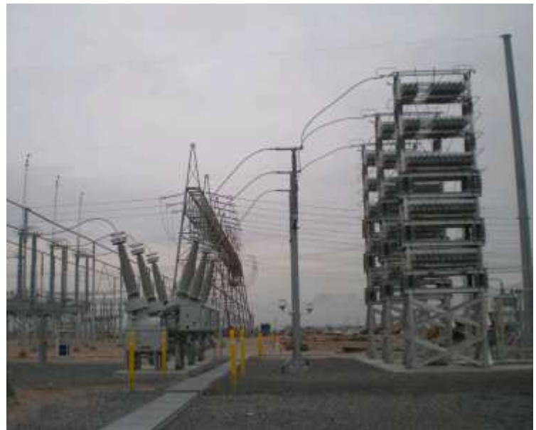
SF 6 gas-filled breakers & capacitor bank (Arn)
