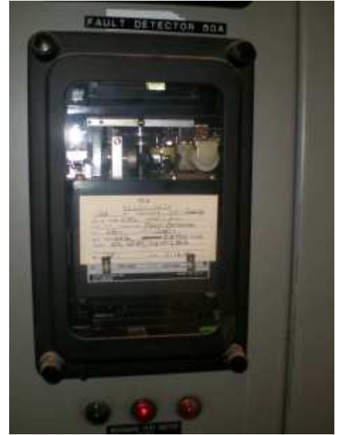
Electromechanical Relay (Arn)
