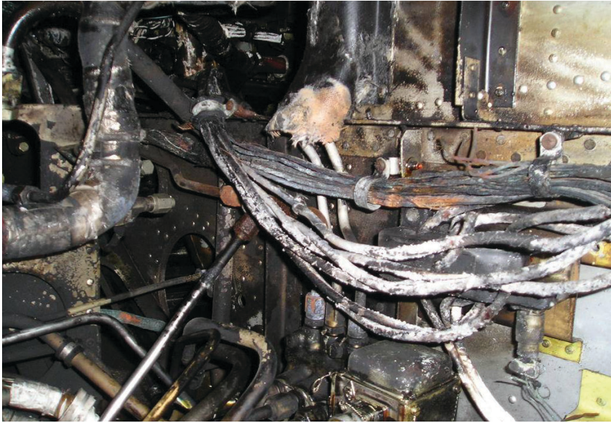
A rat's nest of wiring in the belly of an aircraft at the FAA Test Site, Albuquerque
