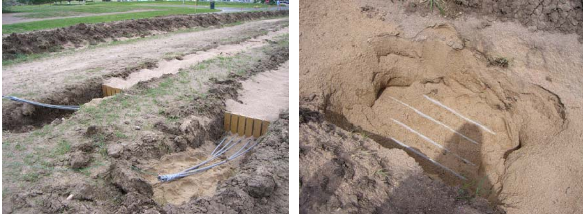
Figure 13 (Left picture) Ends of two anchors extending from trenches 1 (left) and 2 (right), 7' apart. This shows the plywood spacers used to hold the strands approximately 4" apart in the trenches, as shown in the right photo.
