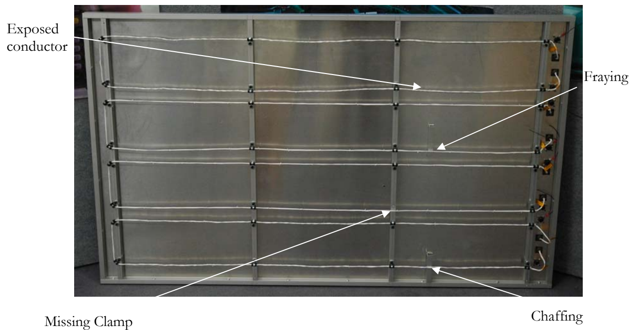
Figure 14 – Test panel 2 harness anomalies.
