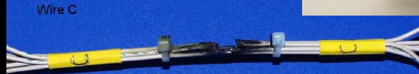
10 A Thermal Breaker Tripped
